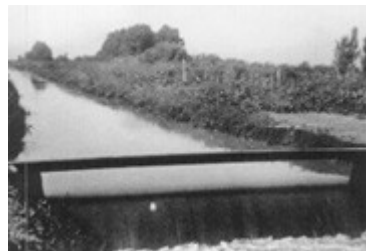
Jordan & Salt Lake Canal looking south at 1100 East 1200 South. Circa 1900.
