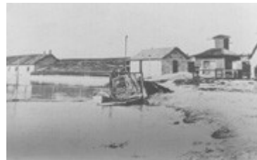
Utah Lake Pumping Plant located at the outlet of Utah Lake in Lehi, Utah. Circa 1901
